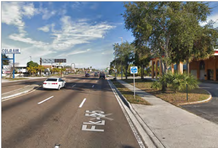
Existing 34th Street N. facing North
