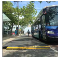
BUS STOP PLATFORMS
