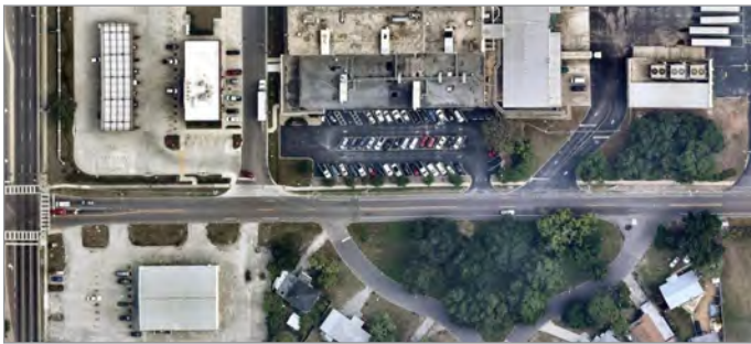
Existing 13th Avenue
