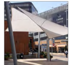
TEMPORARY SHADE STRUCTURE
